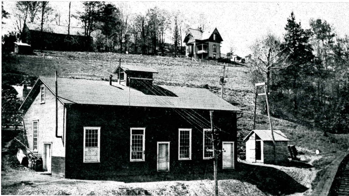
The Dushore Electric Company Plant.
